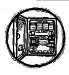
**DO** locate your electrical control panel where it will be protected from potential vandalism and have unobstructed access.
